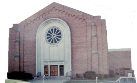
Existing Sanctuary Completed in 1962
